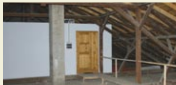
Modular storage block under construction, Csongrád
