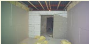
Modular storage block under construction, Museum of Ethnography
